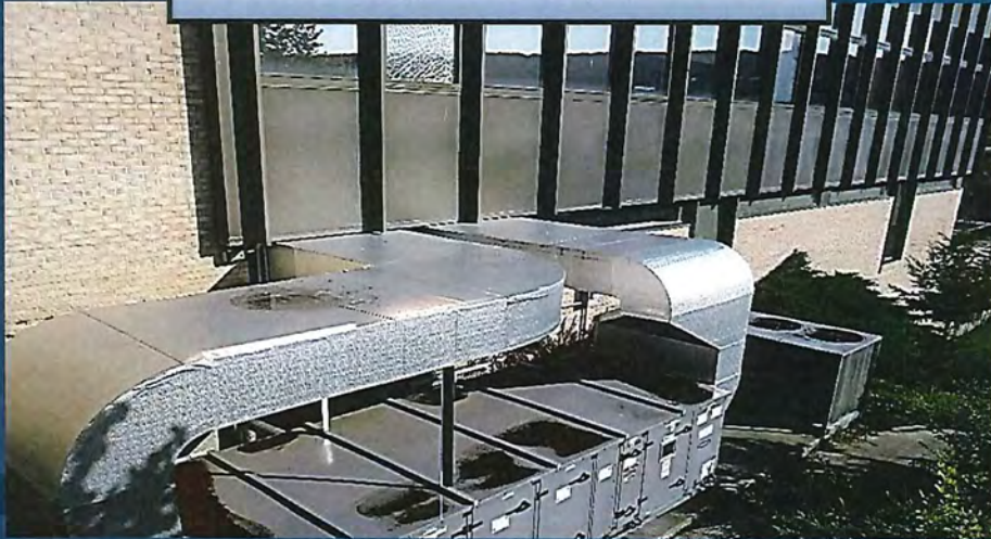
Hinkle Library – Exterior Repair ($3.3 Million)
