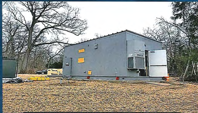
Replace Electrical Substation No. 45 ($1.6 Million)
