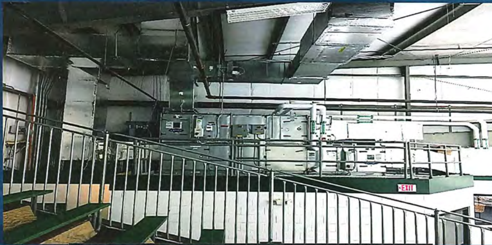
Upgrade Ventilation to Iceplex Building ($1.0 Million)
