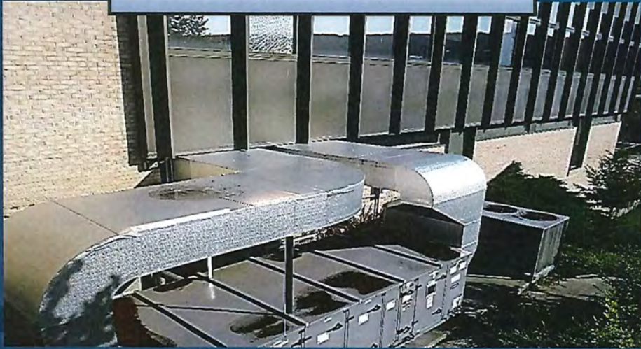
Hinkle Library – Exterior Repair ($3.3 Million)
