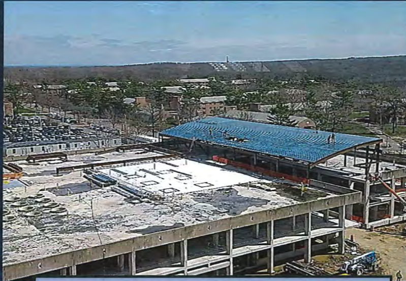
Student Union Rehab ($77.4 Million)
